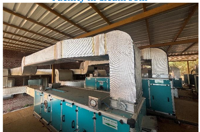
Ventilation systems (HVAC, exhaust fans).
